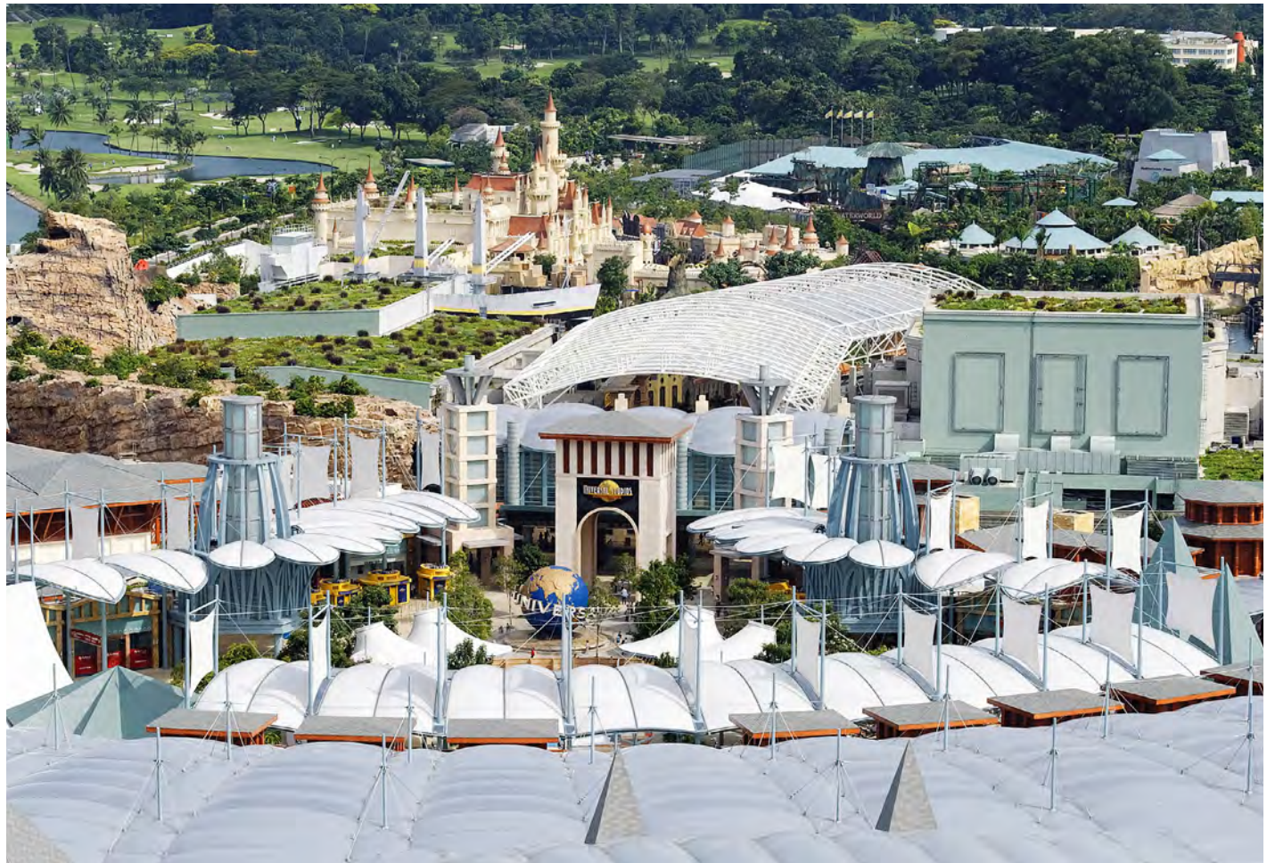
Green roofs and canopy system at Resorts World Sentosa.
